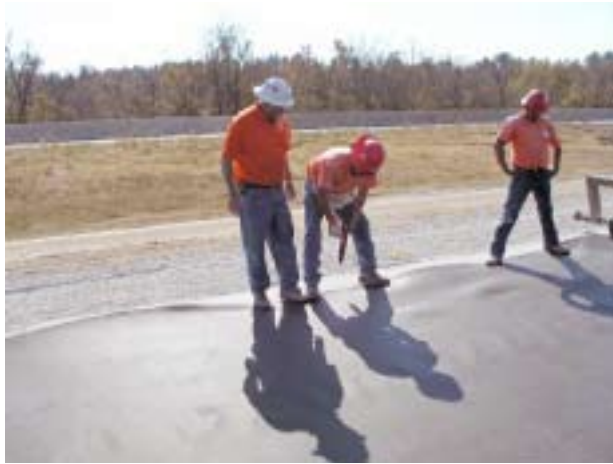
Figure 16. Fastening geotextile to CTB on I-40 project.
