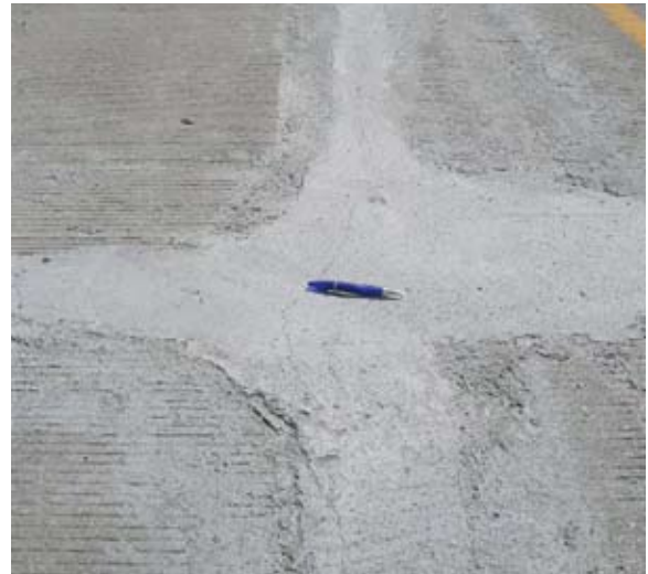
Figure 5. Repair and replacement of damaged concrete with flowable fill.
