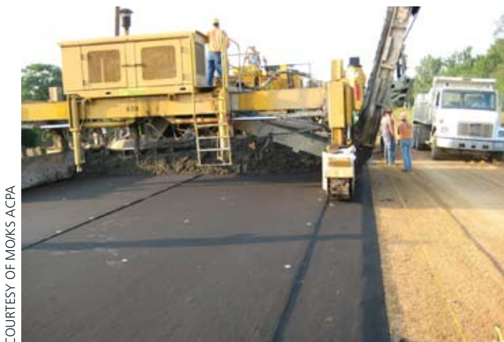
Figure 11. Overlay placement along Route D project.
