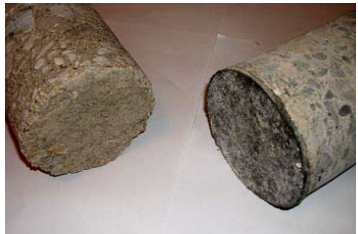
Figure 22. Core of I-40 project showing new concrete bonded to geotextile interlayer (underlying CTB not bonded).
