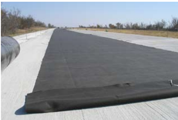
Figure 15. Geotextile installation on I-40 project.
