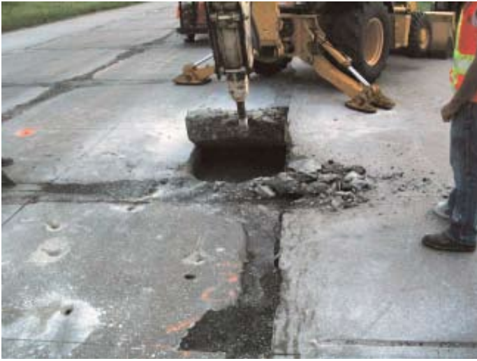
Figure 23. Removal of concrete pavement from a thin nonwoven geotextile in Kansas.
