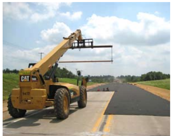
Figure 6. Transport and application of geotextile from rolls along Route D project.
