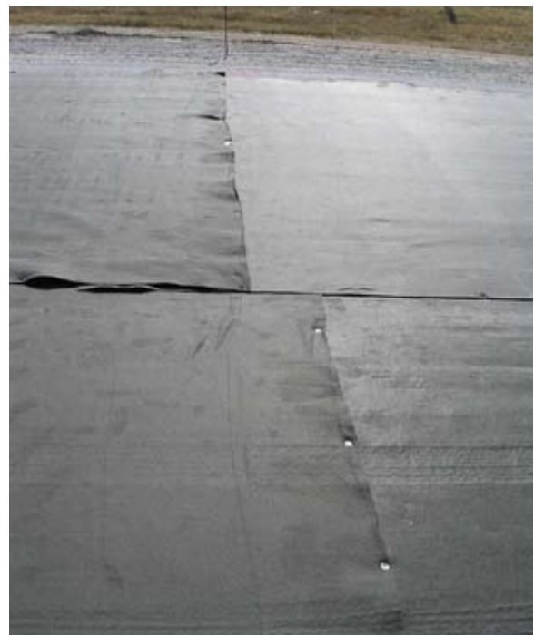
Figure 18. Lapping seams of geotextile on I-40 project.
