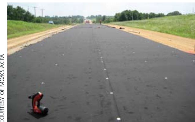
Figure 9. Overlap of geotextile on Route D project.
