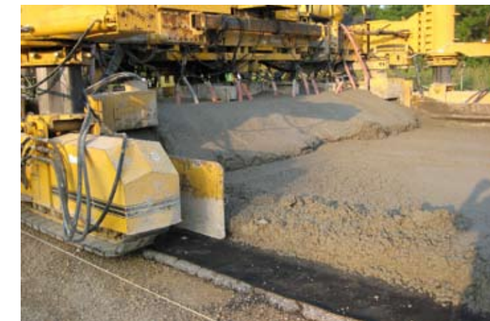
Figure 10. Prewetting of geotextile before paving Route D project.
