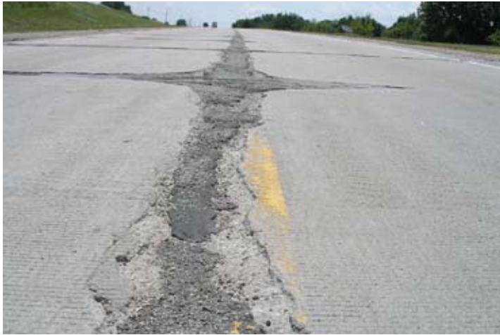
Figure 4. Typical existing pavement condition along Route D before overlay.
