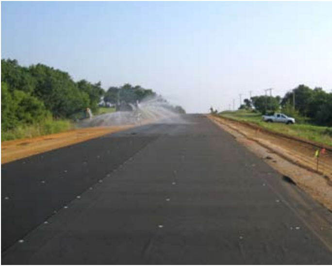
Figure 10. Prewetting of geotextile before paving Route D project.
