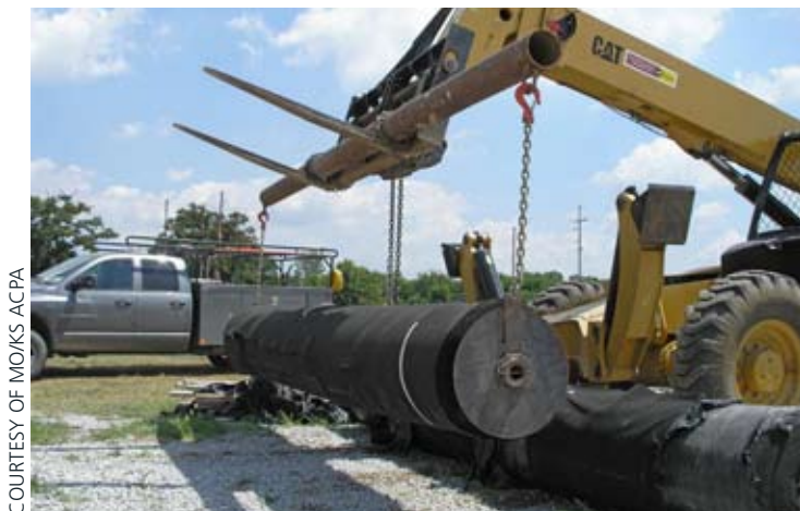
Figure 6. Transport and application of geotextile from rolls along Route D project.
