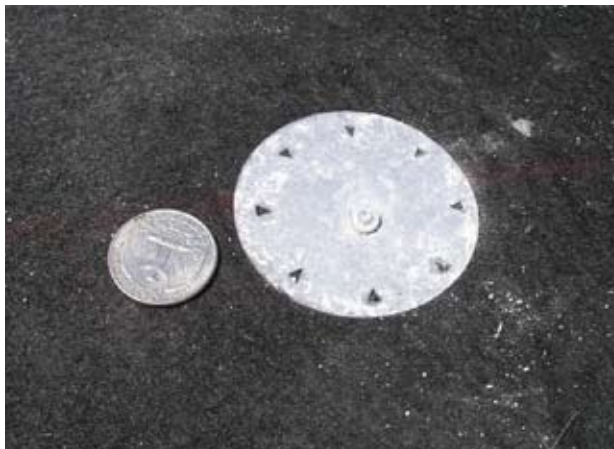
Figure 7. Fastening geotextile to existing concrete pavement along Route D project.
