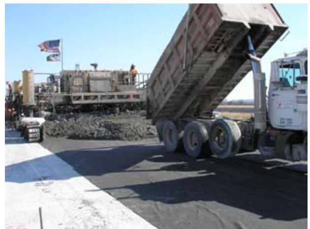
Figure 20. Paving new concrete pavement on geotextile on I-40 project.
