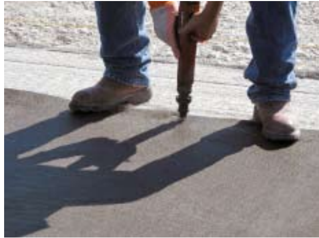
Figure 16. Fastening geotextile to CTB on I-40 project.
