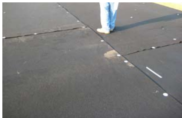
Figure 9. Overlap of geotextile on Route D project.
