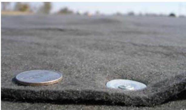
Figure 17. Hilti X-DNI fasteners used on I-40 project.
