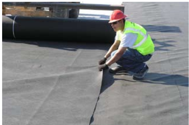
Figure 15. Geotextile installation on I-40 project.
