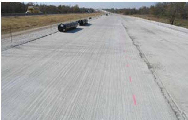
Figure 14. Delivery and installation of geotextile rolls on I-40 project.
