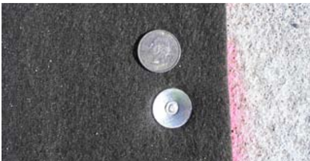
Figure 16. Fastening geotextile to CTB on I-40 project.
