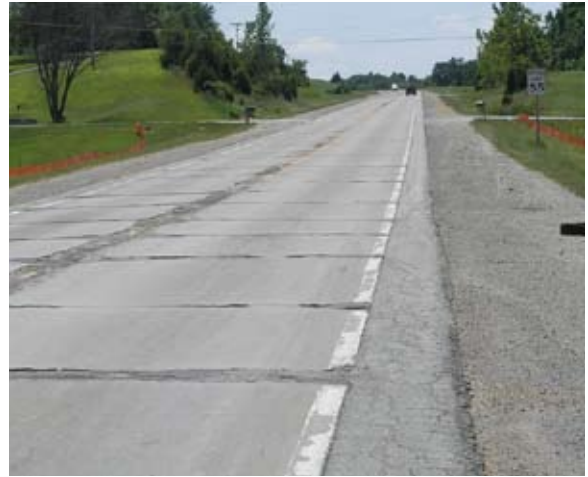
Figure 4. Typical existing pavement condition along Route D before overlay.
