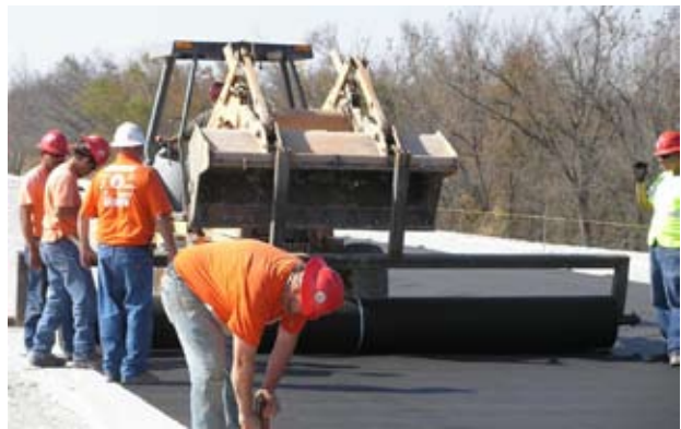
Figure 14. Delivery and installation of geotextile rolls on I-40 project.
