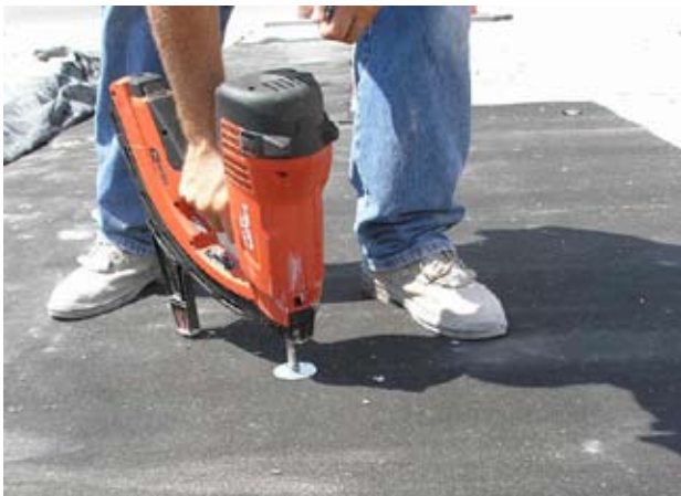
Figure 7. Fastening geotextile to existing concrete pavement along Route D project.
