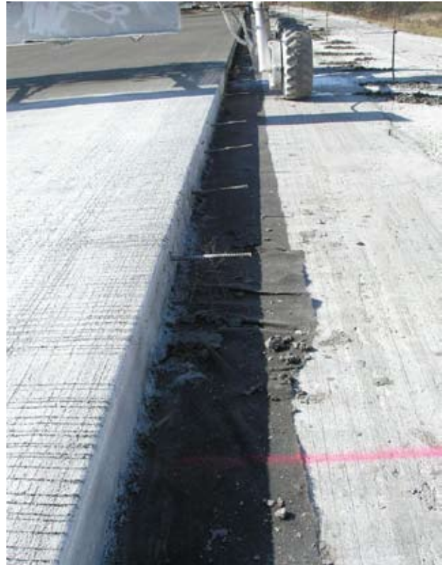
Figure 21. Geotextile terminating under shoulder on I-40 project.
