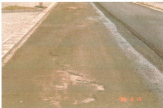
Figure 6. - Surface after milling
