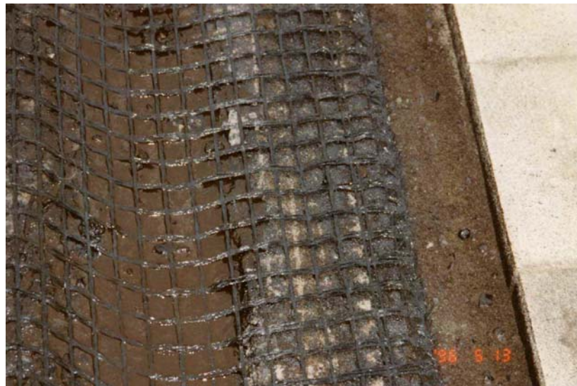
Figure 6. Difficult spots during installation
