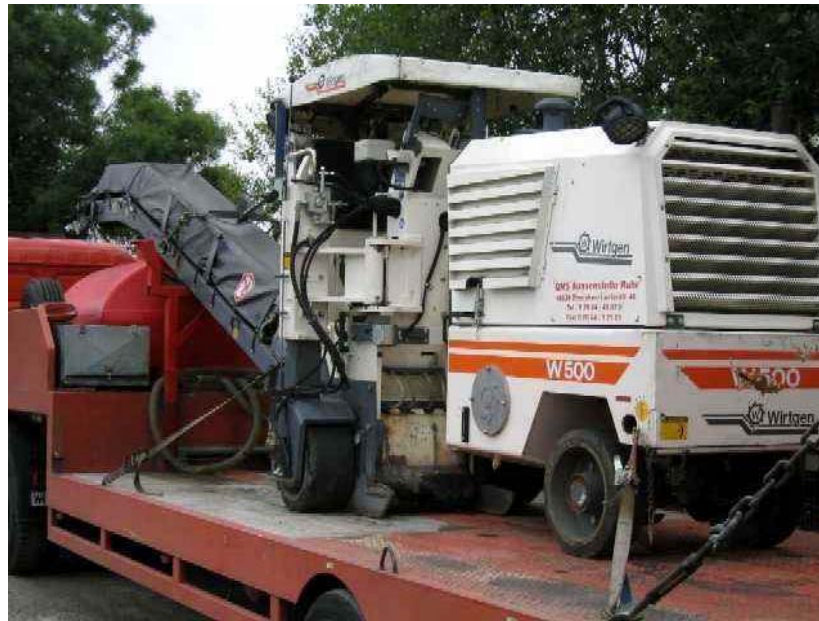
Figure 9. Milling of reinforced asphalt
