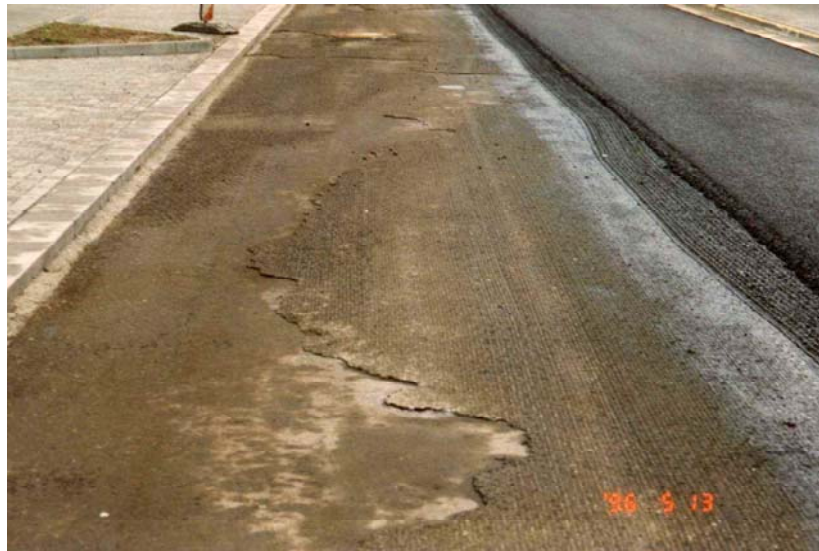
Figure 5. Surface after milling
