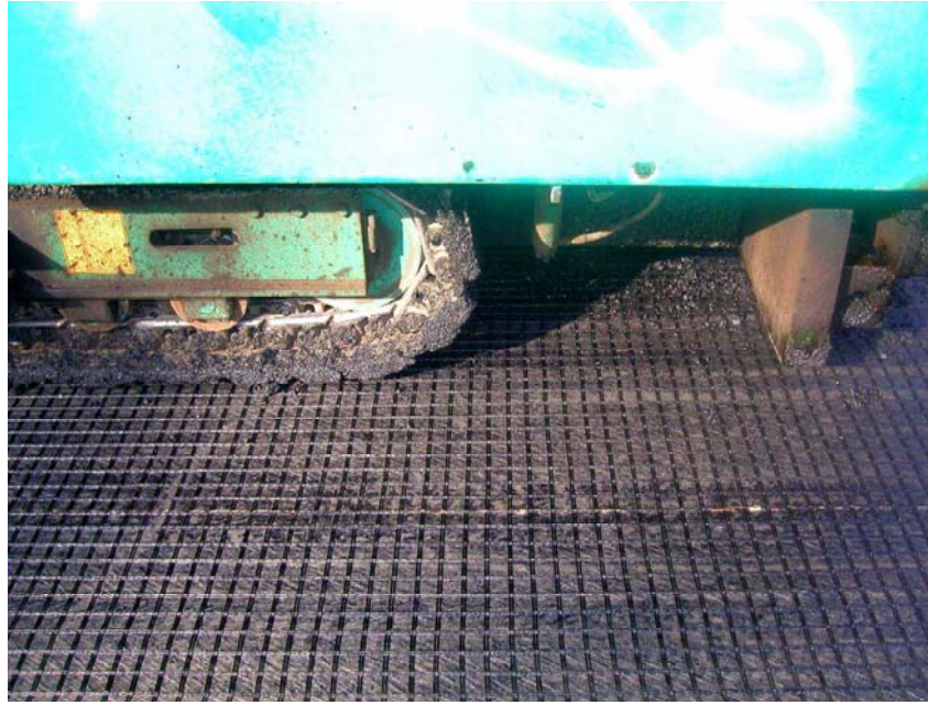
Figure 7. HaTelit® C 40/17 trafficked by a tracked paver
