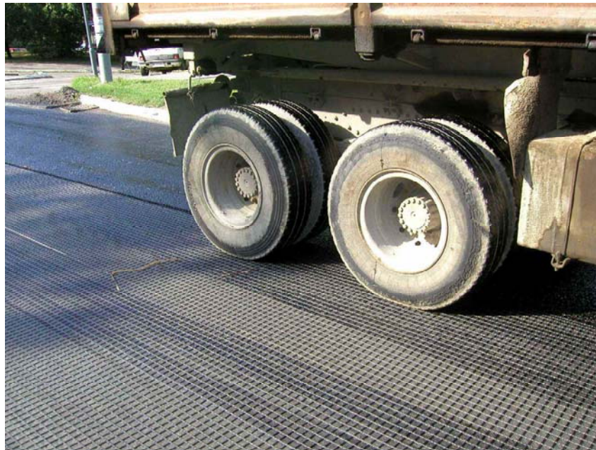
Figure 8. HaTelit® C 40/17 trafficked by a blacktop lorry
