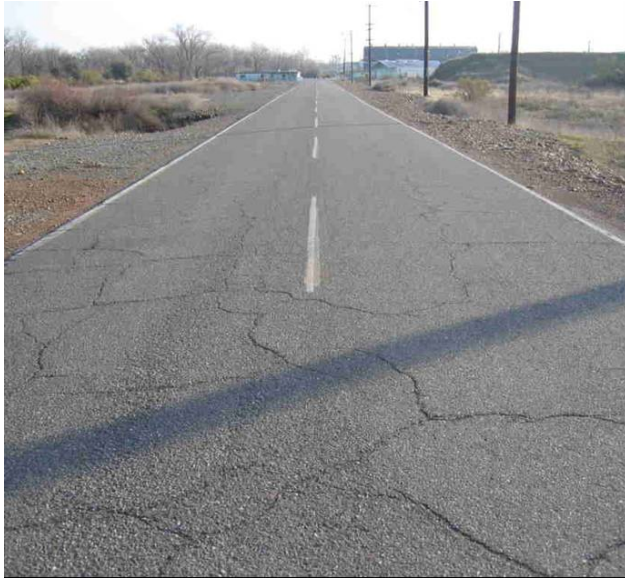
Figure 2 Aerojet Facility, Northern California 20-year old 2-inch hot mix asphalt overlay (Brown, 2003)
