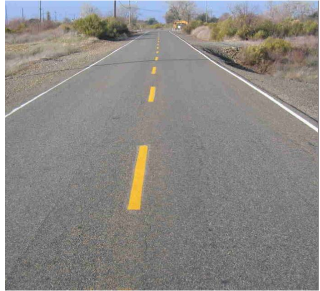
Figure 3 Aerojet Facility, North California 20-year old double chip seal over fabric (Brown, 2003)
